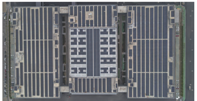
The images are of solar panel installations at the Company's Shenzhen, China and Tianjin, China locations.
