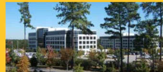
Lenovo Morrisville, NC, USA site
